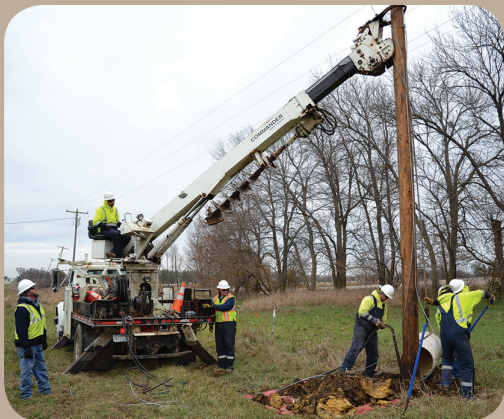
Lineworkers from Legacy Contracting, Inc. out of Minnesota continue to replace poles along Hwy. 14 near Greene. Legacy is completing FEMA work for us that will continue into the spring of 2018.
