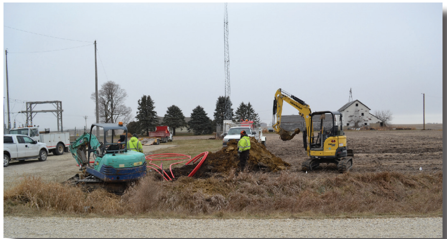
Trenchers begin work for Butler County REC's new solar array, Solar II, located north of the town of Bremer.
