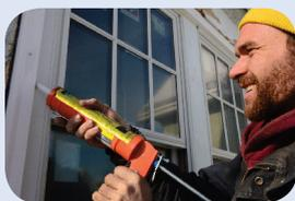
The area should be dry before you apply the new caulk. Apply the caulk in one continuous stream, and make sure it sticks to both sides of the crack or seam. Use a putty knife to smooth out the caulk, then wipe the surface with a dry cloth.
